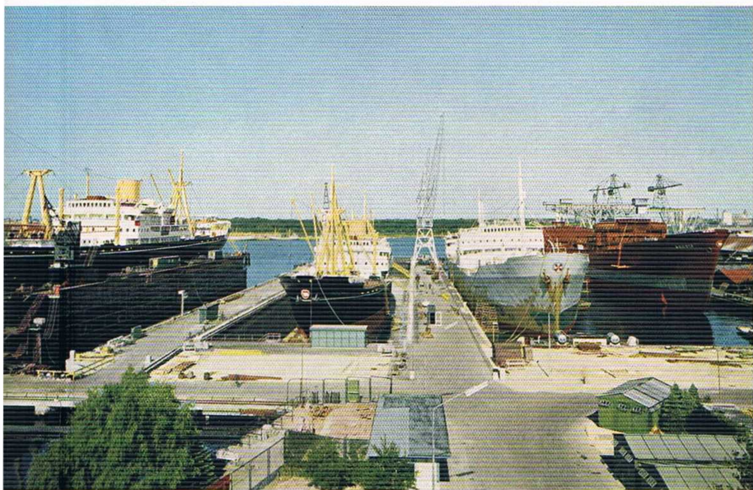
View of a small section of the shipyard area, showing in the centre the newest 38,000 tons dw. dry dock.
