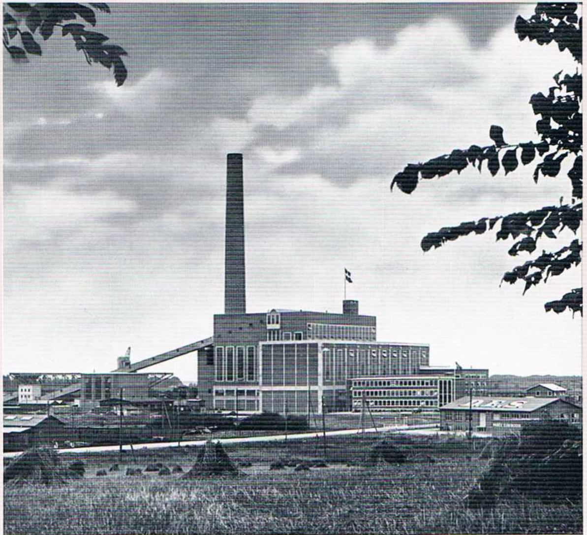
The Funen Power Station at Odense, Denmark.
